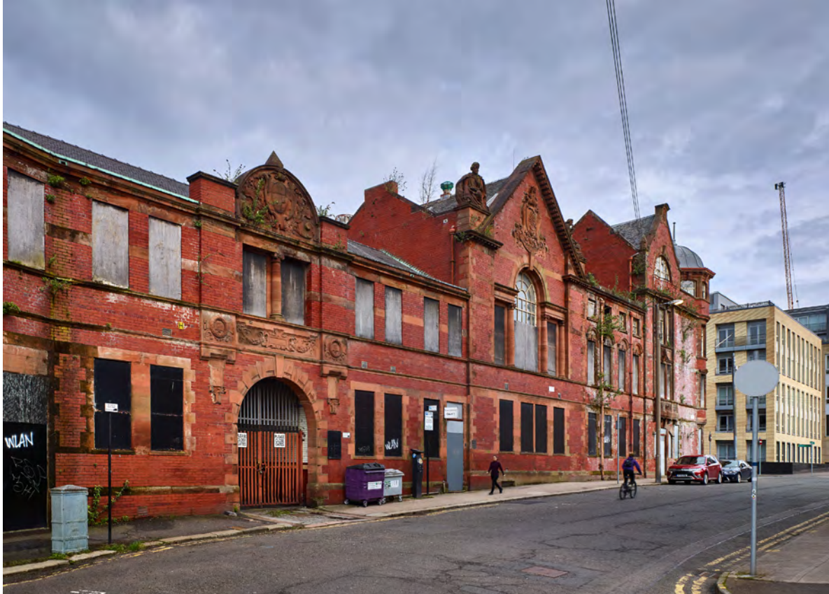
Existing View from Turnbull Street
