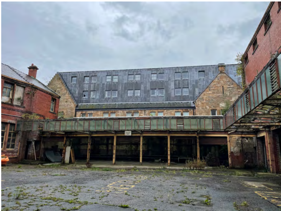
Existing view from internal Court Yard
